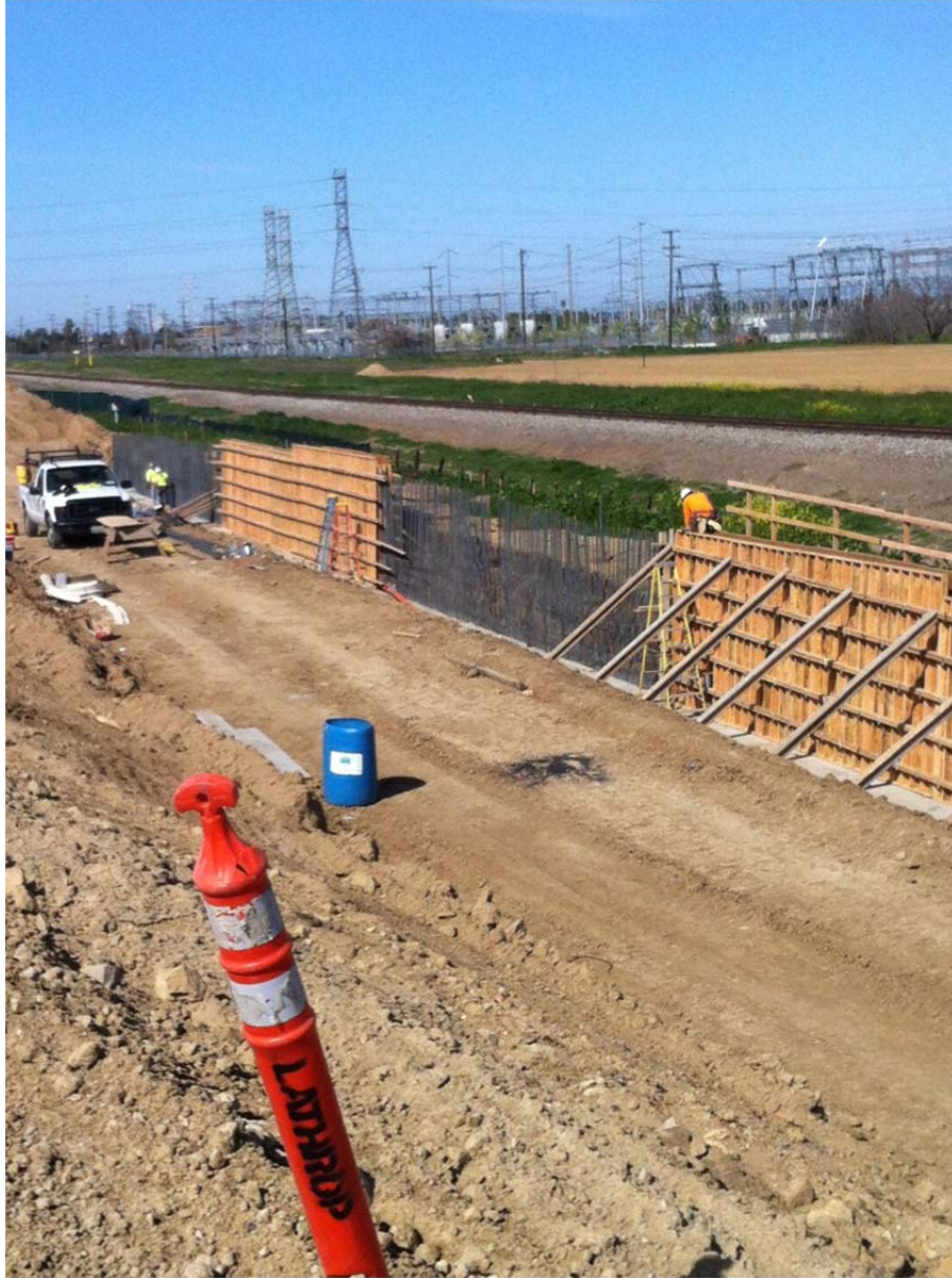
February 27 , 2013. Antioch Station Parking. Construction of Retaining Wall.
