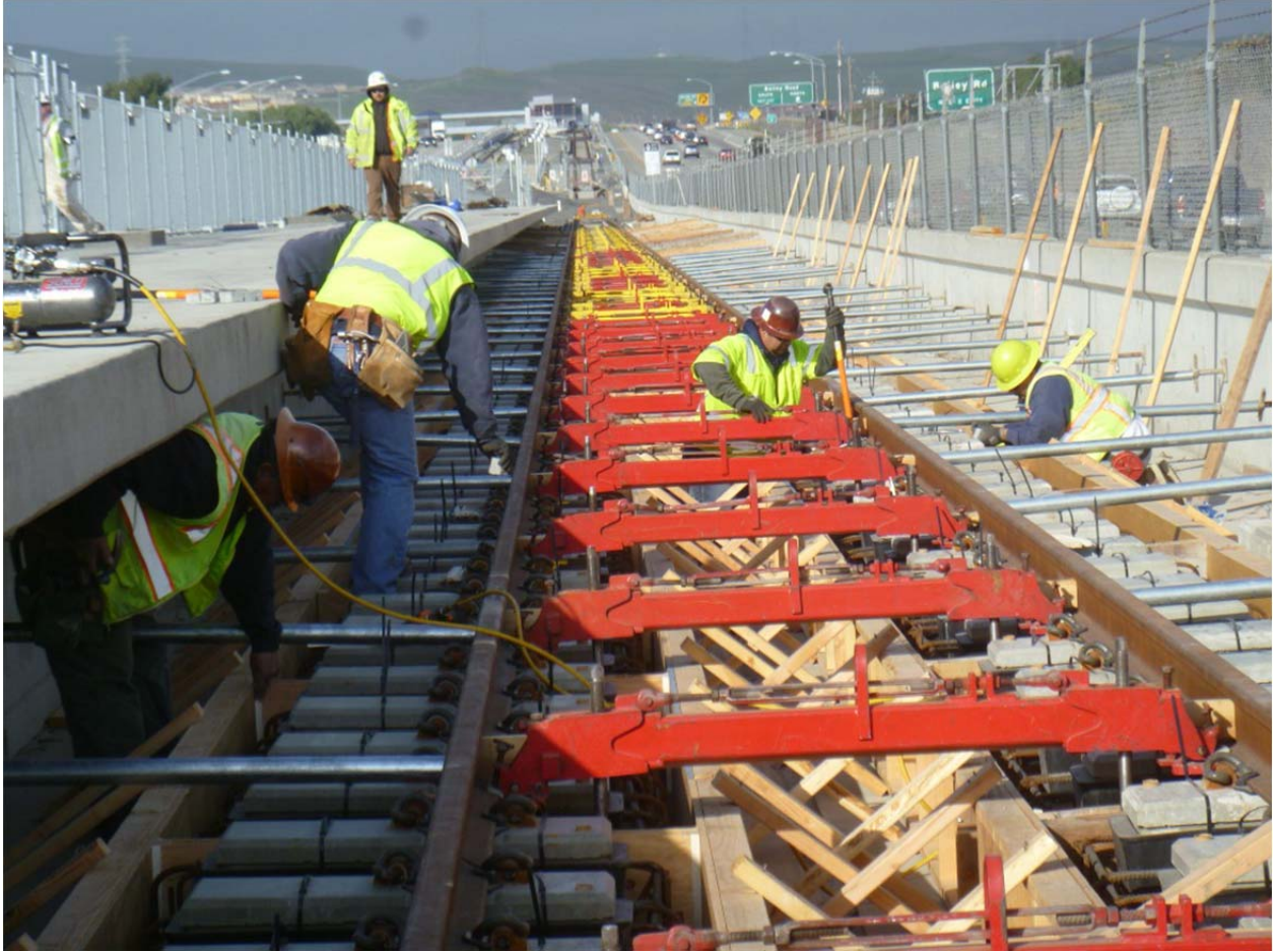
March 4, 2013. eBART Transfer Platform. Rail Installation For BART Vehicles.
