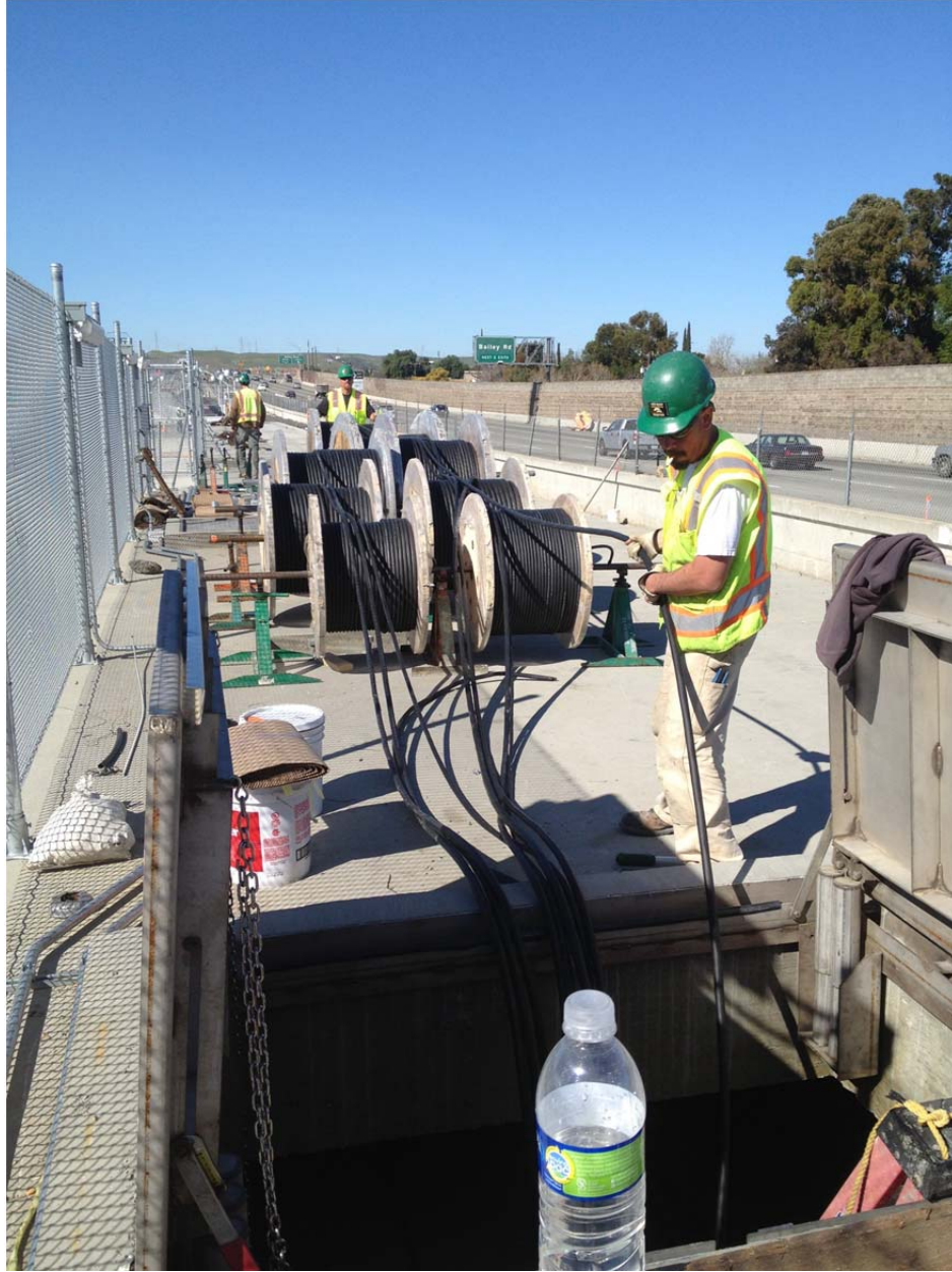
March 1 , 2013. Transfer Platform. Train Control Cable Installation
