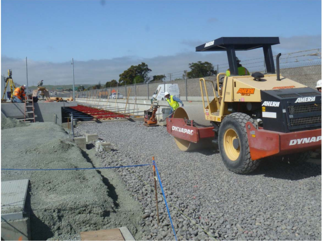
March 4, 2013. Transfer Platform. Track Ballast Installation
