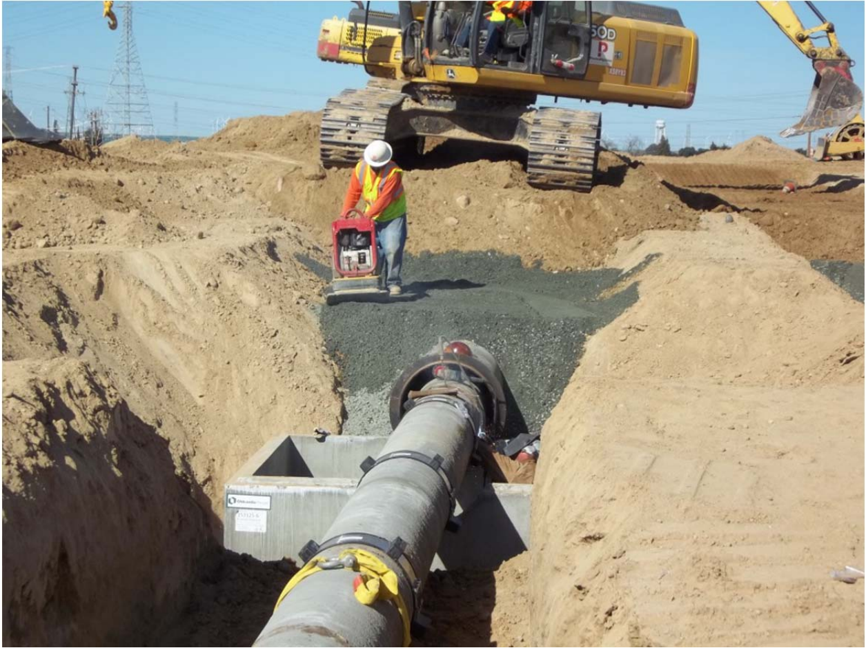
March 4 , 2013. Antioch Station Parking. Water Line Installation.
