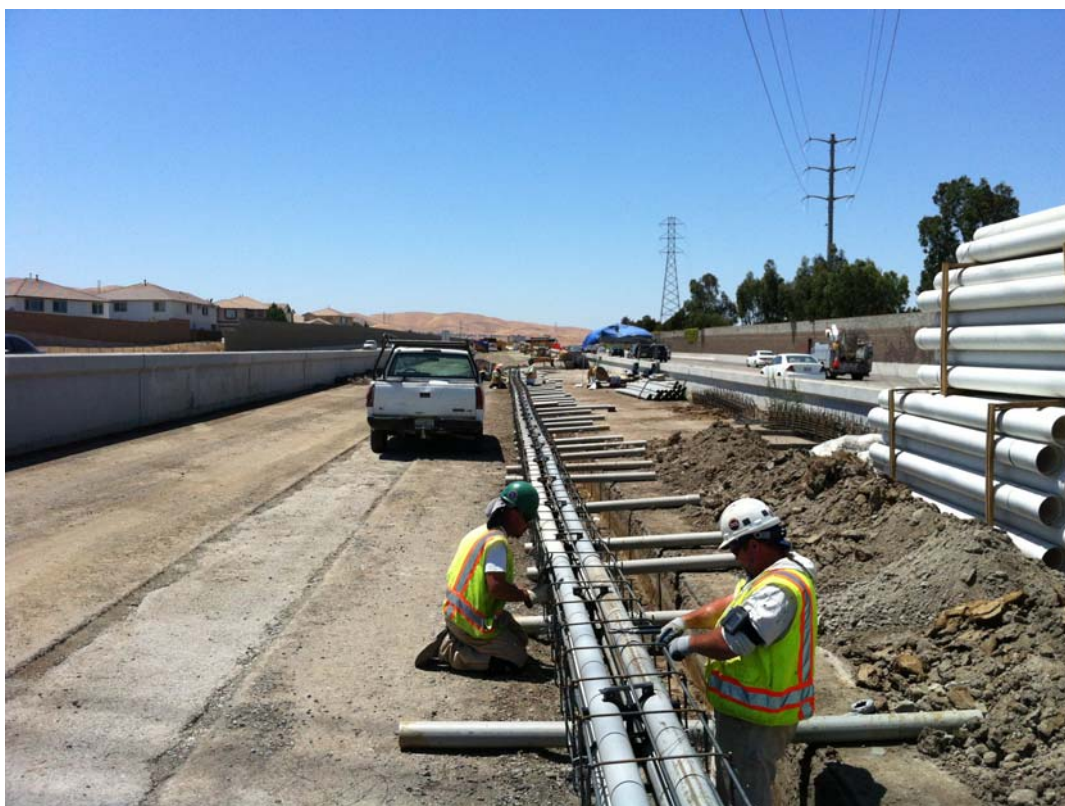
July 25, 2012. Installation Of Reinforcing Steel Cage for Electrical Duct Bank
