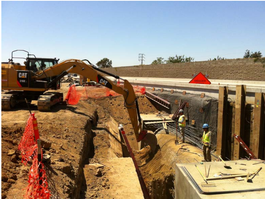
July 24, 2012. Excavation Of Next Segment of Mokelumne Aquaduct
