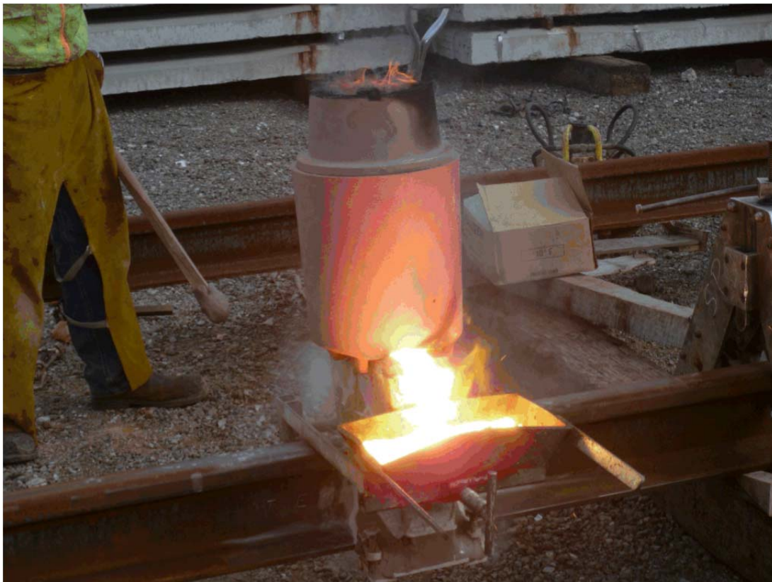
02/05/13 eBART 04SF-110A Rail Welding
