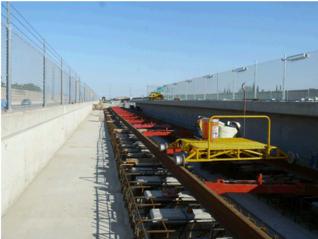
02/06/13 eBART 04SF-110A. Installation of Rail at Transfer Platform
