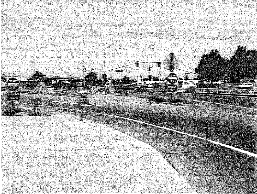
Photo 6. The actual pedestrian crossing. Pedestrians routinely cross the ramp here, rather than use the tunnel. There is no crosswalk, no traffic signal or stop sign; motorists have a “free right” to come down the ramp and merge onto Bailey Road at high speed if they can. Yet pedestrians still choose to cross here rather than use the tunnel.
