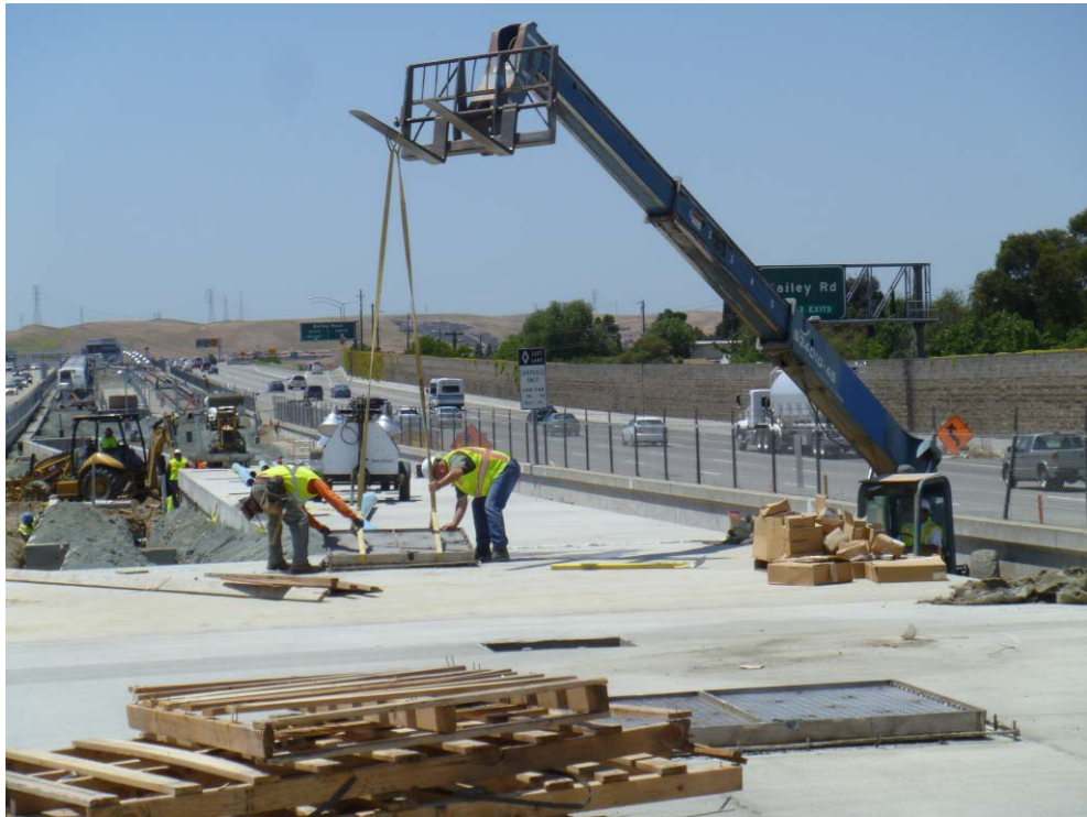
Installation Of Access Hatches. Transfer Platform. May 29, 2012.
