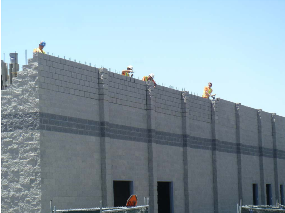
Completing CMU Block Installation. Ancillary Building. May 29, 2012.
