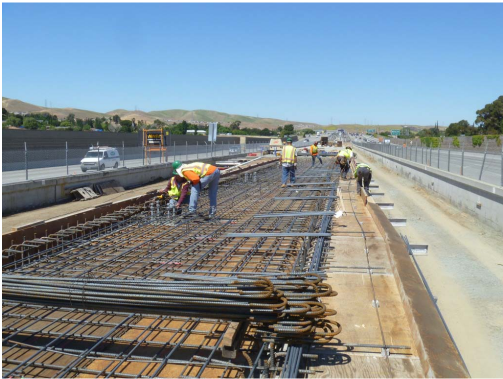
Reinforcing Steel Installation At Transfer Platform. May 23, 2012.
