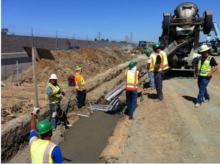
Encasement Of Communications And Power Ductbank. June 1, 2012.
