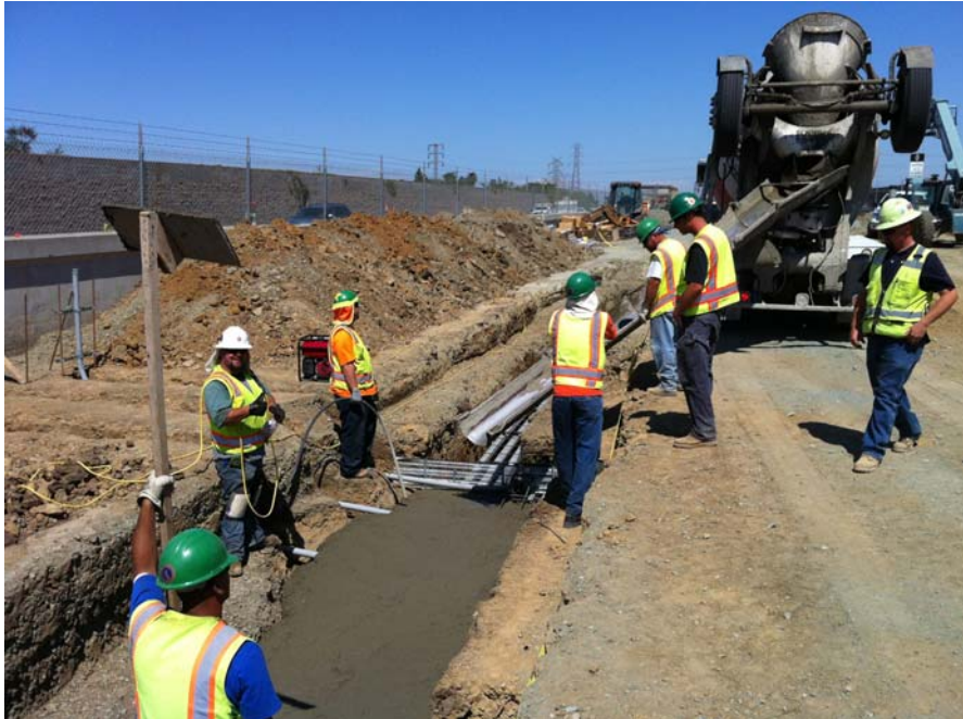
Encasement Of Communications And Power Ductbank. June 1, 2012.
