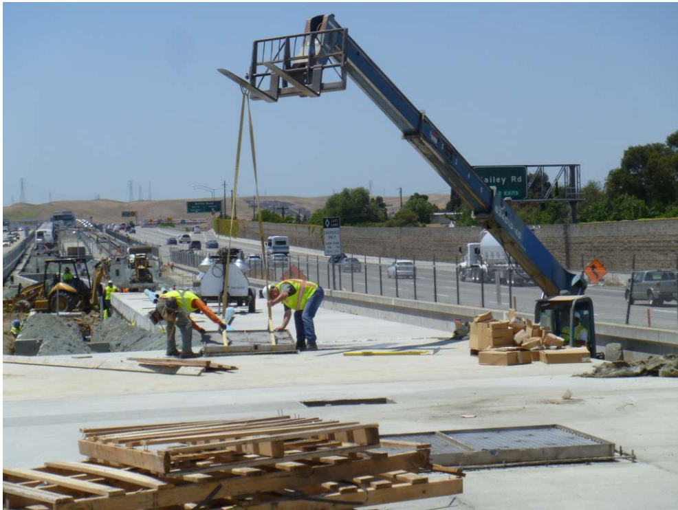
Installation Of Access Hatches. Transfer Platform. May 29, 2012.
