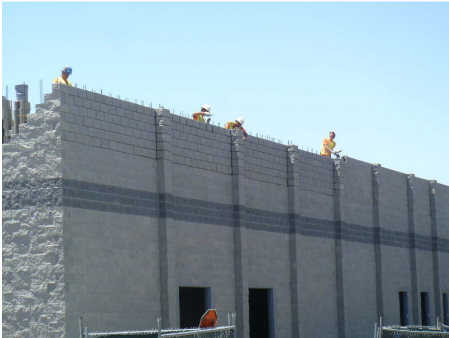
Completing CMU Block Installation. Ancillary Building. May 29, 2012.
