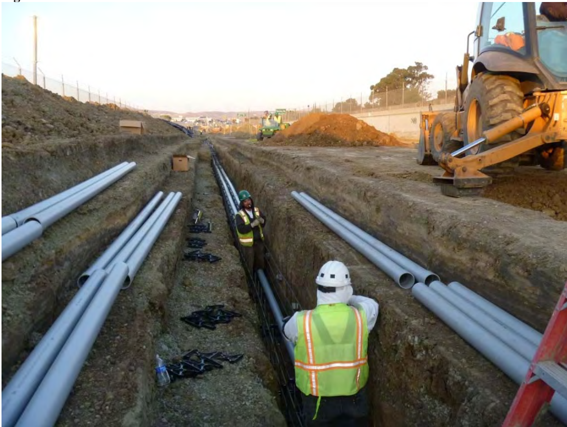
Figure 2: Duct Bank
