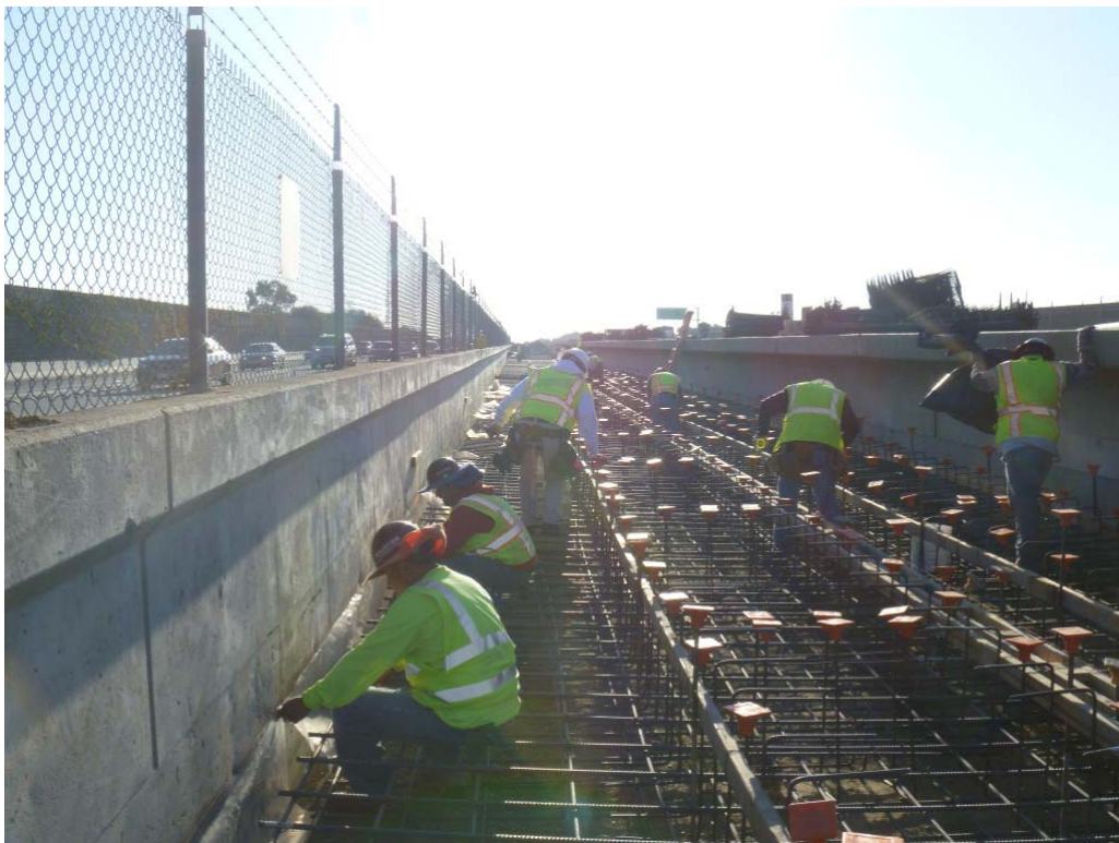
Sept. 4, 2012. Track Slab Work Adjacent to BART Platform.
