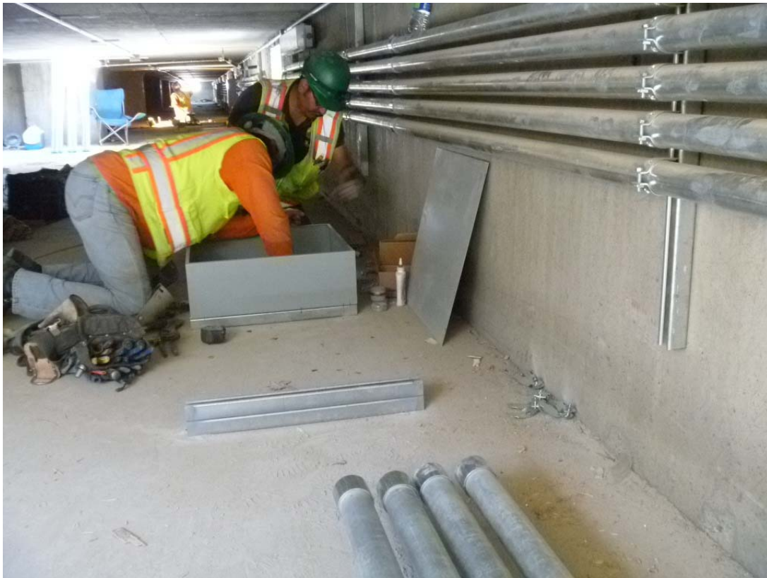
Sept. 4, 2012. Electrical Work. Under platform Space.
