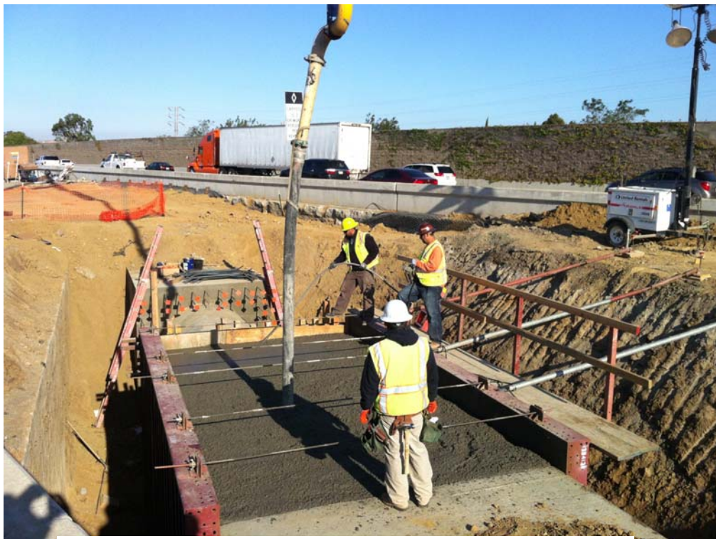
Sept. 6, 2012. Placement of Concrete. Mokelumne Aqueduct
