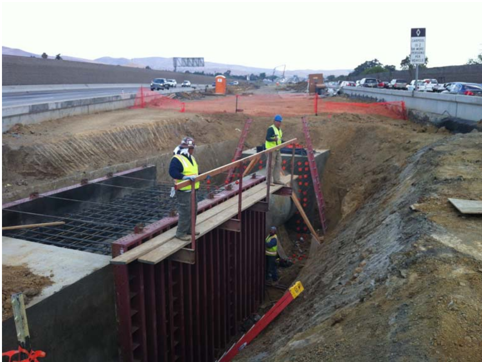
Sept. 5, 2012. Preparing Forms for Mokelumne Aqueduct Concrete
