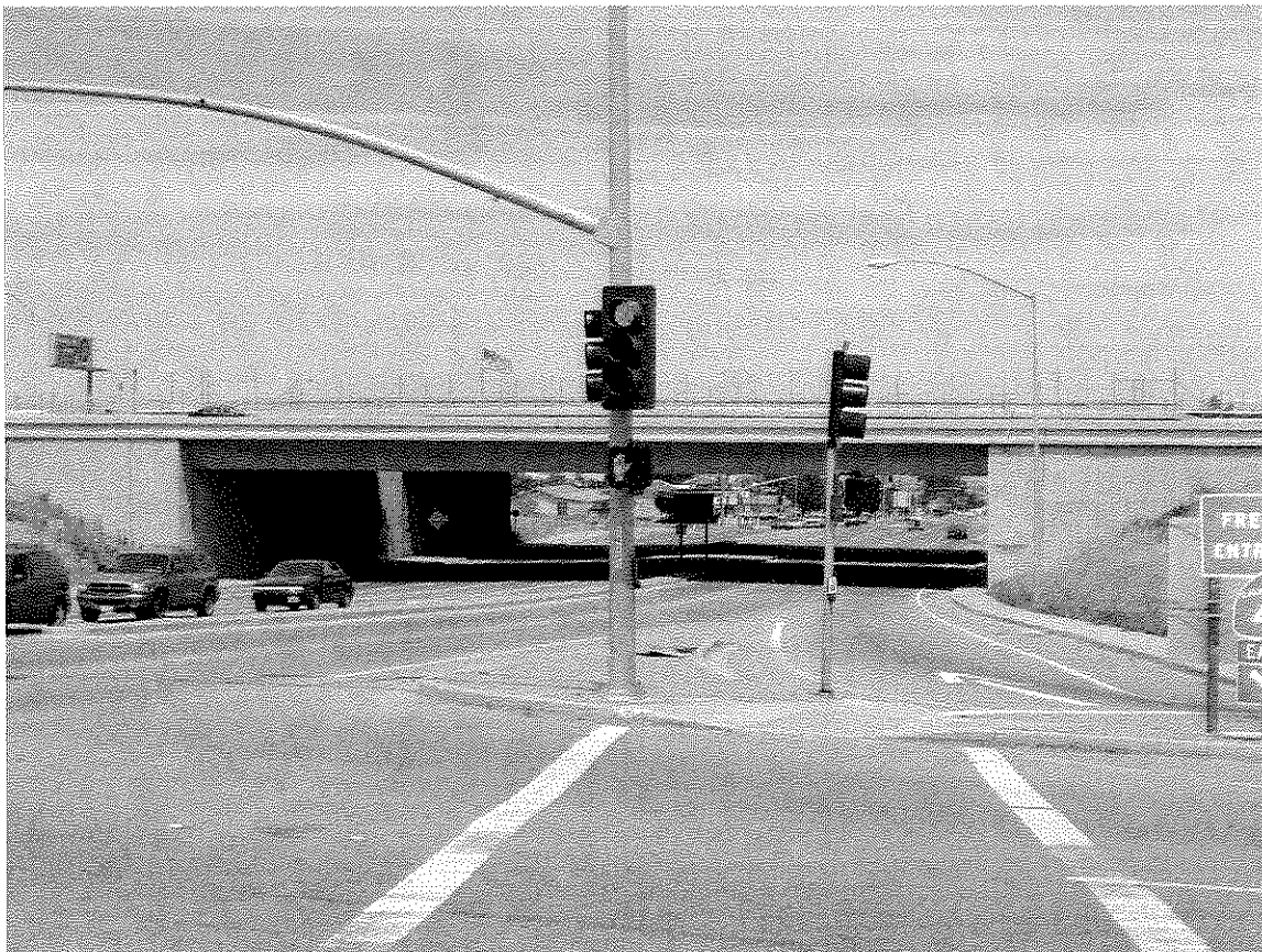
Photo 7. Looking north along Bailey Road toward the freeway overpass. The little “porkchop” island in the foreground provides the only safe haven for bicyclists and pedestrians who have to travel across two ramps – first the on-ramp (foreground) and then the off-ramp (beyond the island). The speed at which vehicles come down the off-ramp, and relatively small size of the island, make an uncomfortable atmosphere for pedestrians and bicyclists waiting on the island to cross the next ramp.
