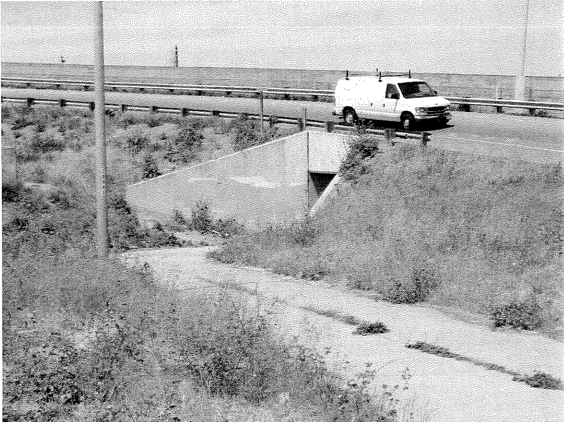
Photo 4. The other side of the tunnel. The photograph shows the sloping walkway leading from the tunnel to Bailey Road. The slope makes it difficult for those with mobility problems to use it. The condition and secluded nature of the tunnel makes it unappealing to all pedestrians and bicyclists. As mentioned earlier, County staff has yet to see a pedestrian use this tunnel for pedestrian purposes.
