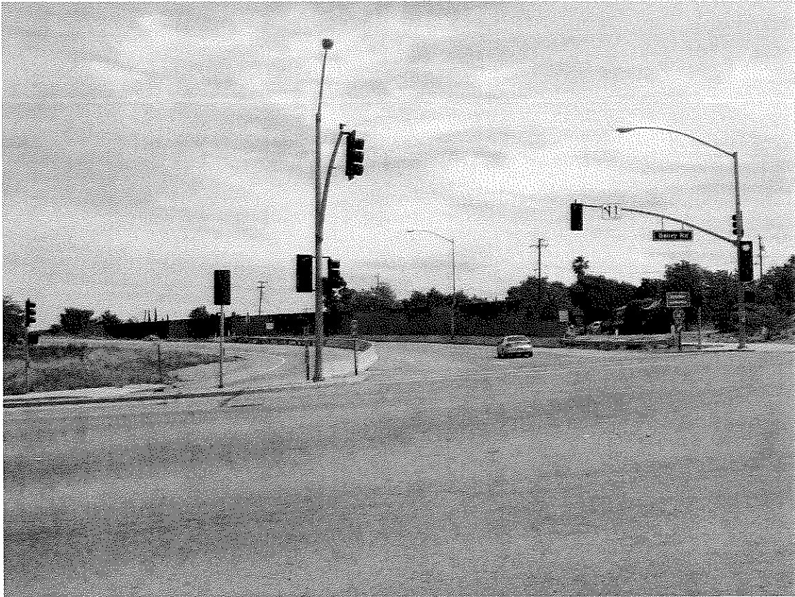
Photo 1. Looking across Bailey Road to the eastbound freeway ramps. A bicyclist or pedestrian traveling north along Bailey (which would be from right to left in this photo) must cross these two freeway ramps, first the on-ramp and then the off-ramp. Both ramps have vehicles making quick right-turns onto or off of the ramp. (All of the photographs in this grant application were taken between 12:15 p.m. and 1 p.m. on a weekday, when there isn't much traffic on the freeway ramps.)
