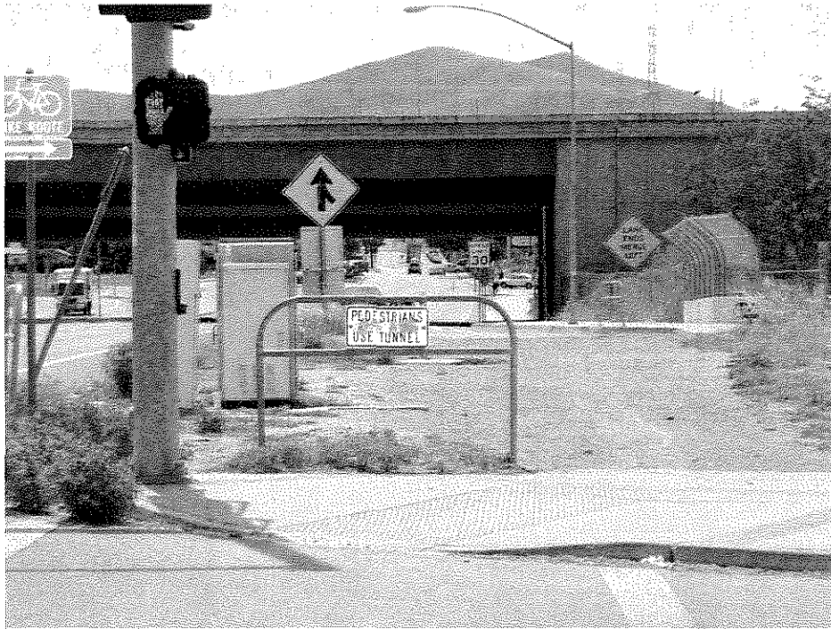
Photo 2. Looking south along Bailey Road toward the freeway overpass. Pedestrians and bicyclists traveling south along Bailey Road to get to the Pittsburg/Bay Point BART Station are directed by the white sign to walk to the right, along the sidewalk, and use a concrete pedestrian tunnel to go under a freeway off-ramp. Virtually all pedestrians walk straight across the dirt rather than using the pedestrian tunnel.
